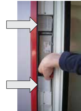
Take out dirty filters and put new filters back in. Put cover back on and screw on.
