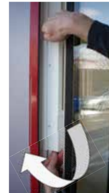
Pull the sash slightly closed and tilt the cover towards the outside when taking it off.
