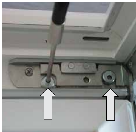
Turn security bolt on both tilt hinges with 5mm Allen key by 180°.
