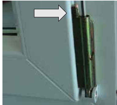
Raise or lower sash with 4mm Allen key.
