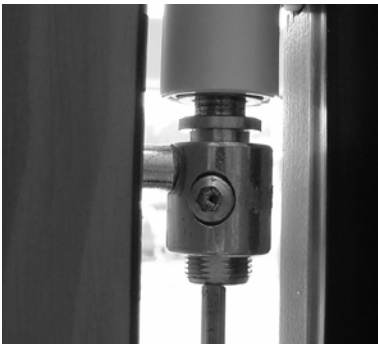
Bring adjustable support to desired height by turning to the left or to the right and correct the other hinges too.
