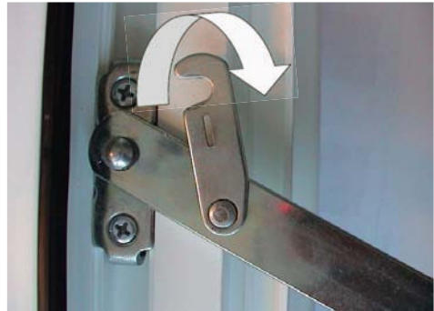
2. Horizontal adjustment Unlock and unhinge cleaning stay-arm. ATTENTION: Sash is now unsecured and must be secured by a second person! Tilt sash no more than 90°!
