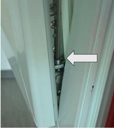
Vertical adjustment Version a Tilt sash. Raise or lower sash with 4mm Allen key.
